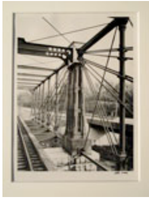
Railway Trestle Bridge ©David Schaffer
