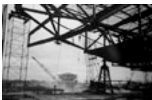
"Building Skeletons, New York's World's Fair Construction" ©Arthur Lavine, 1963
